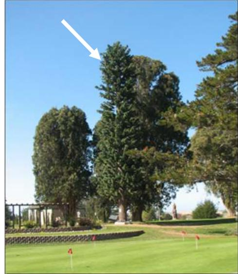
Illustrative example of a tower camouflaged as a tree ("alternative tower structure")
